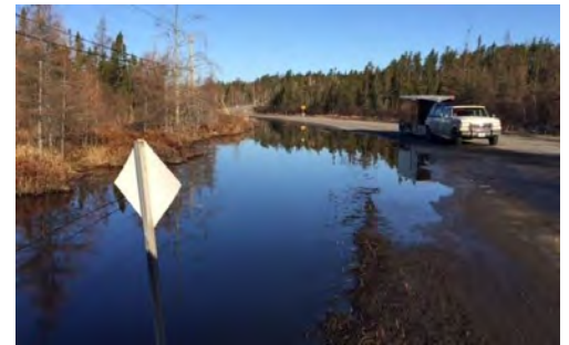
This road in Northern Ontario floods every spring, leading to closure. Photo from https://www.cbc.ca/news/canada/sudbury/hwy-537-mto-rehabilitation-1.4573211
