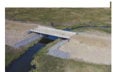
Permanent crossing over creek: Government of NWT.
