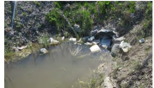
Damaged or blocked culverts and ditches can't carry water away like they should.
