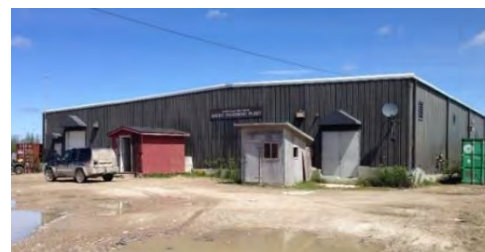
Water treatment plant in Attawapiskat.
