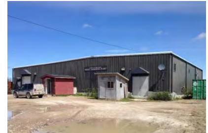
Attawapiskat water treatment plant.
