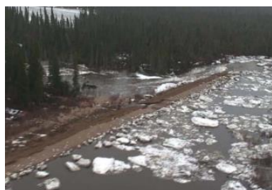
Dyke along the Albany River, South Channel 1
